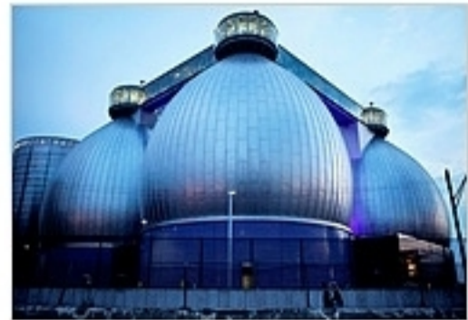
Damon Winter/The New York Times The Newtown Creek Wastewater Treatment Plant in Greenpoint, Brooklyn, is the largest of New York City's 14 treatment plants.
